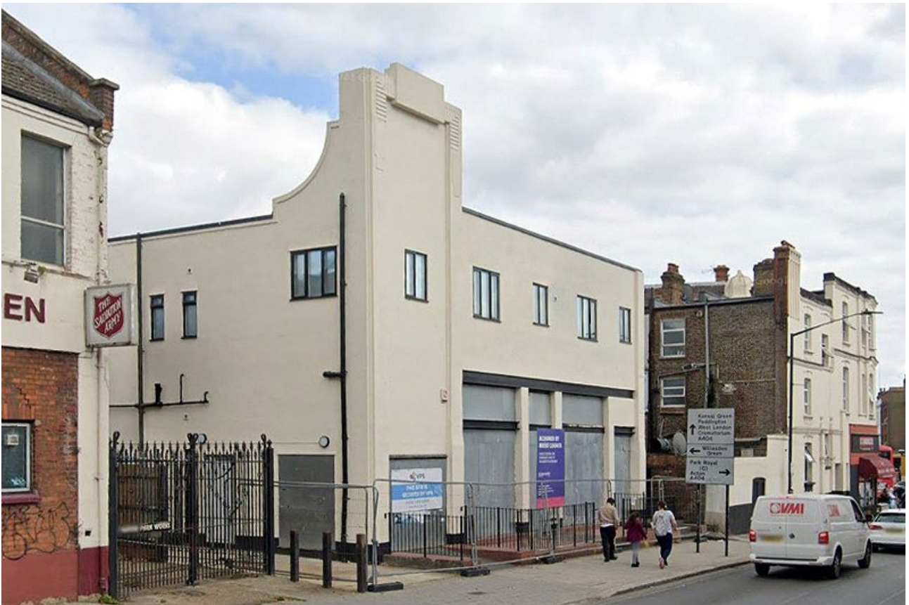
28. Front facade of the former cinema on Manor Park Road.
