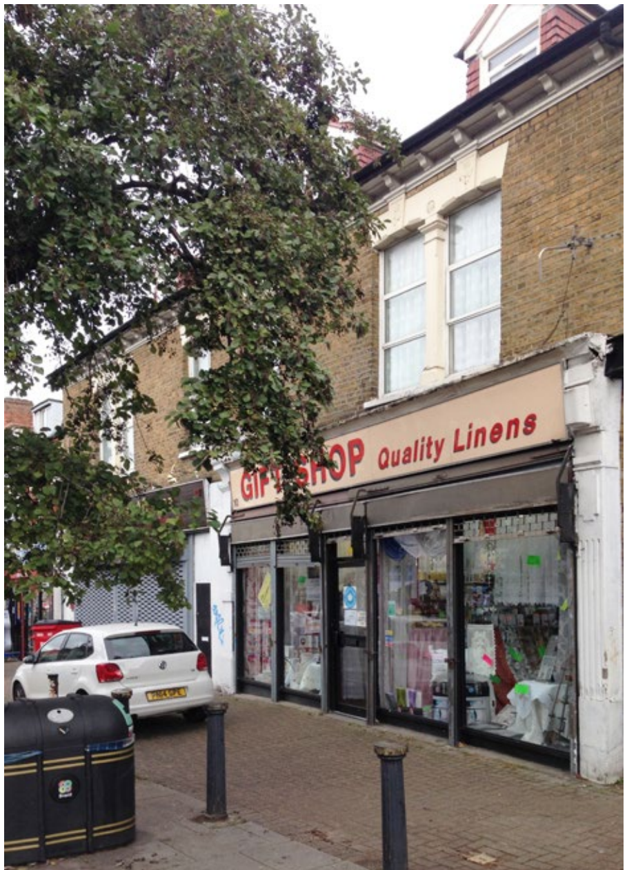
16. The pavement on the east side of Craven Park Road outside no. 10.
